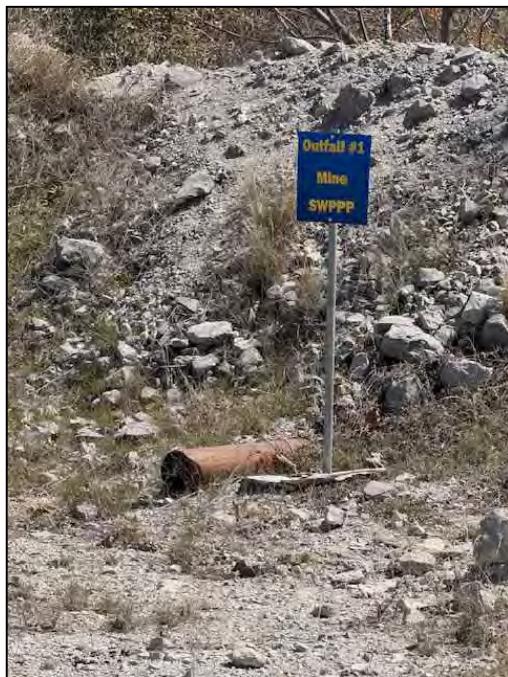
DISCHARGE PIPE FROM HOLDING POND
