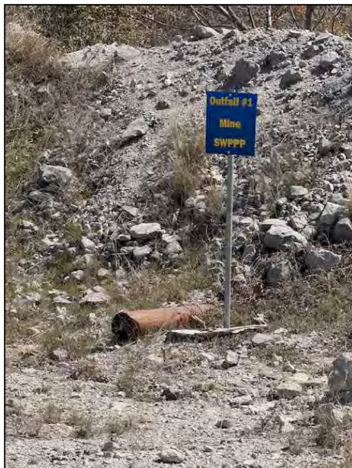
DISCHARGE PIPE FROM HOLDING POND
